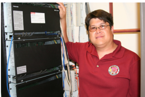
Kevin Shives of Yavapai-Apache Nation relies on the Toshiba Strata CIX670 VoIP system and its additional networked Toshiba Strata CIX systems to support more than 230 users on a mix of IP and digital telephones. He uses Toshiba's eManager to remotely manage the entire system.
